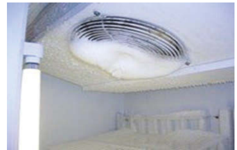
Figure 1 Frozen Refrigerator Coil
